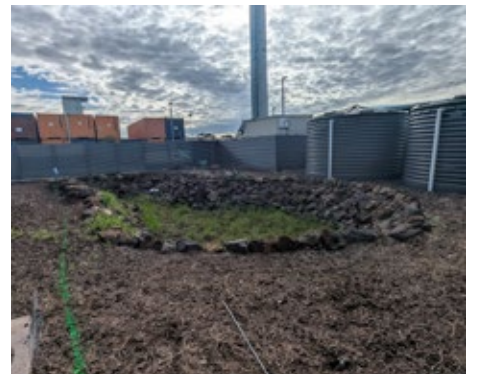
Orana Netley back garden during works
