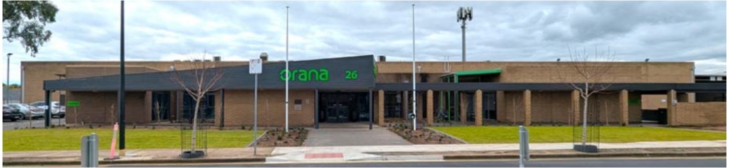
Orana front entrance Watson Avenue after
